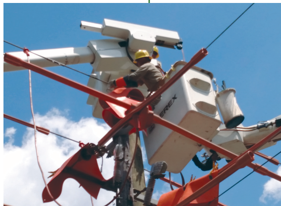
Linemen Jimbo Hammock and Jason Johnson are up in the clouds doing pole change-outs.
